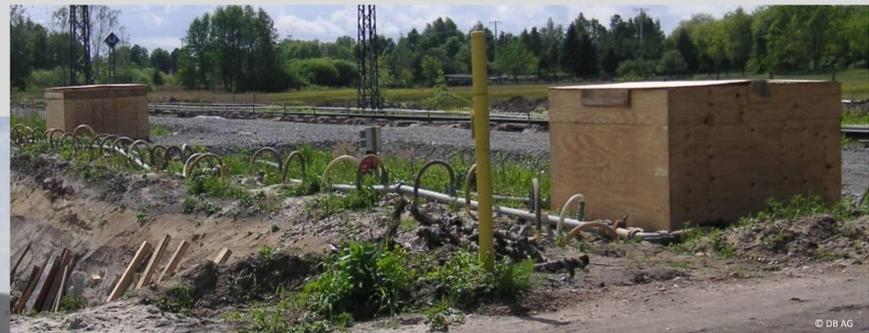
Construction project "Kreuzungsbau Elsterwerda": The vacuum pumps, which operate twenty-four-seven, were encapsulated with insulated wooden enclosures to reduce the construction volume.
