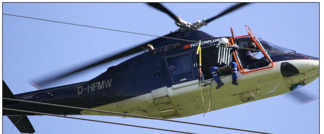
Figure 6: Bird markers are subsequently mounted onto ground cable. Distance between deflectors is roughly 25 m. Photography © S. Ehlers (BIA)
